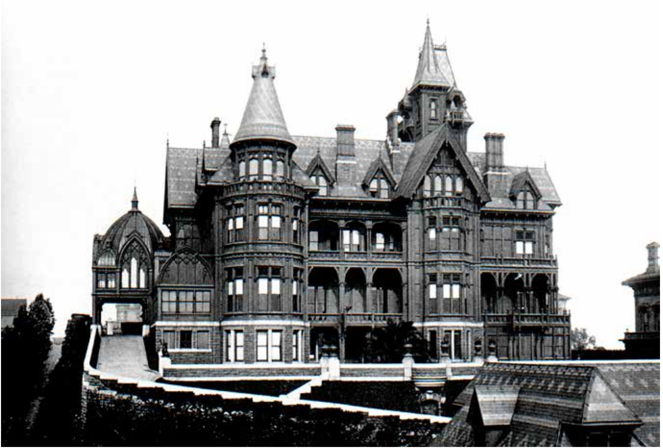
Rear view of the Mark Hopkins San Francisco residence. Photograph courtesy of Ron Henggeler.
